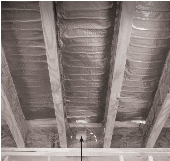
Connect mats at junction box(es).
