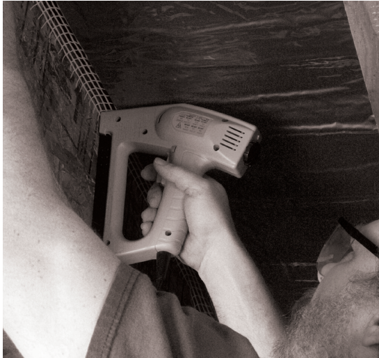
Roll out and staple mat to the floor joists.
