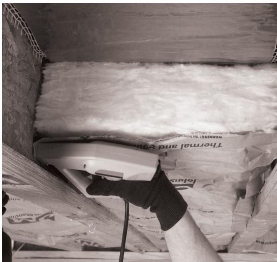
Install insulation.
