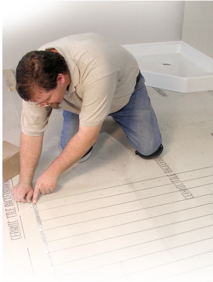
MasterHeat in thin-set mortar over slab
