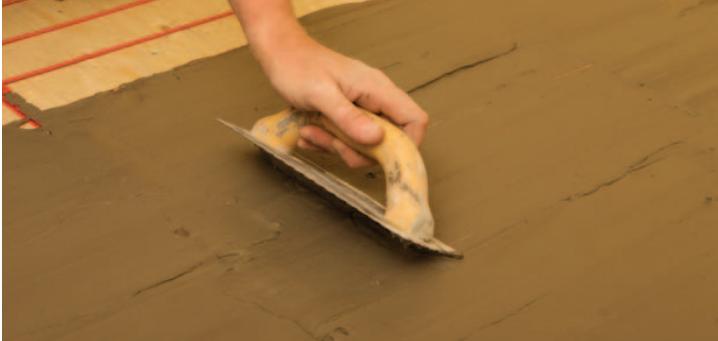
FIGURE 2.52: Thinset mortar method
