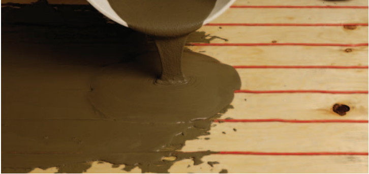
FIGURE 2.42: Self-leveling compound method
