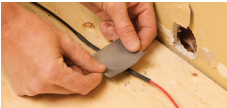
FIGURE 2.23: Secure the cold lead to the subfloor
