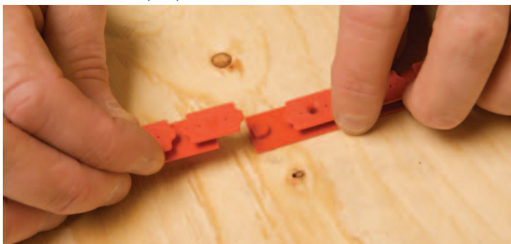
FIGURE 2.25: Snap together Nuheat Cable Guides
