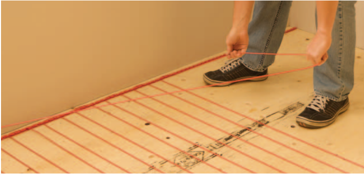
FIGURE 2.27: Install the heating cable
