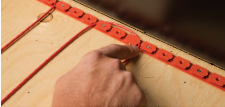
FIGURE 2.26: Install the heating cable
