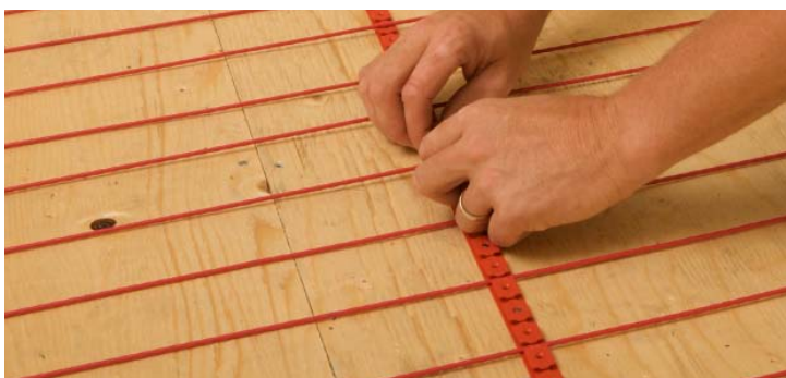
FIGURE 2.29: Install stabilizing guides
