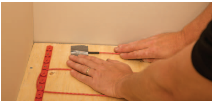
FIGURE 2.28: Secure the end seal
